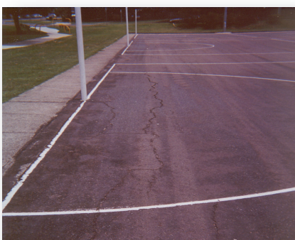
Cracked Asphalt/Hardcourt
